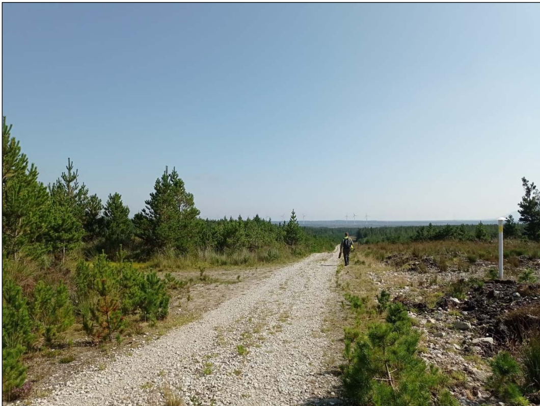
Photo 2: Existing access track along gas pipeline wayleave
